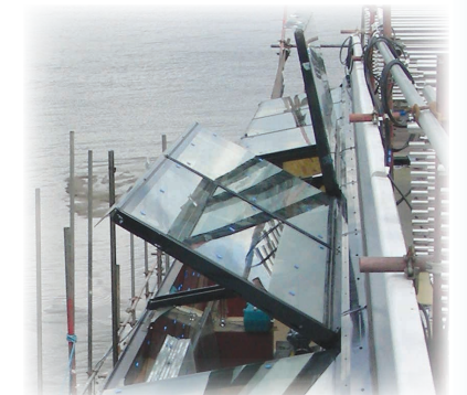
Hydraulically powered opening roof windows
