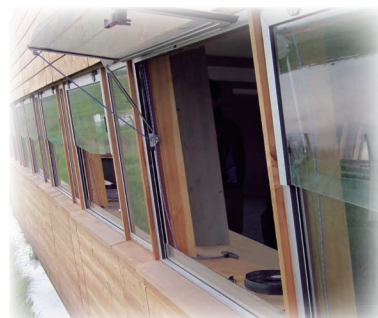
Hide windows comprise of a lower sliding panel and an overlapping upper hinged pane
