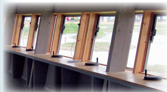
Interior view of the hide, showing the window winders which control the sliding lower panes
